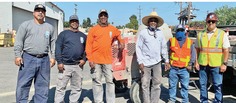
City of Los Angeles Street Lighting Division, members working on this crew are L to R- Danny Hernandez, LeKeith Mackson, Cortez Adams, Alfred Johnson and Business Representative Thony Sarmiento.
